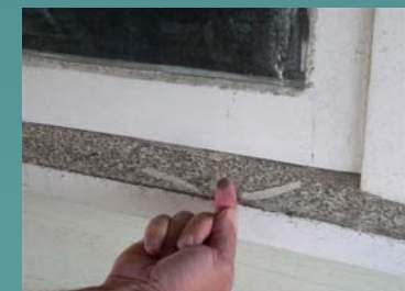
Airborne Pollution on local property from existing Highway
